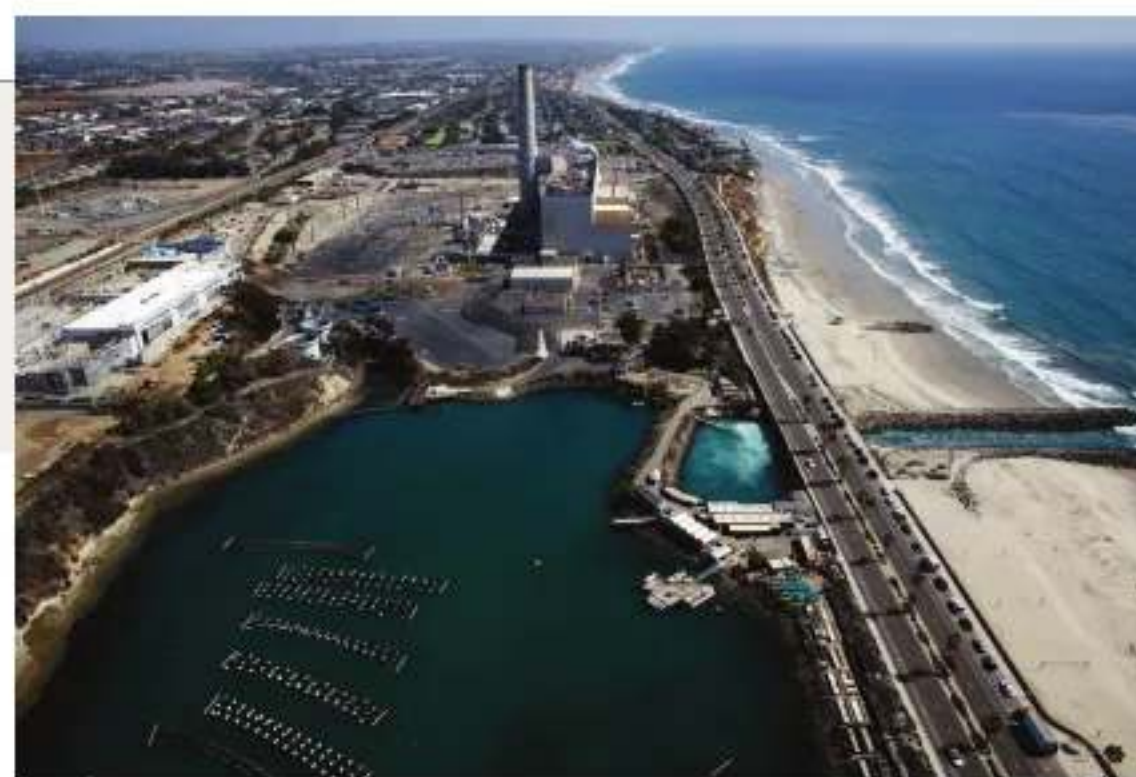
Desalination plants such as this one can produce millions of liters of fresh water from seawater every day.
