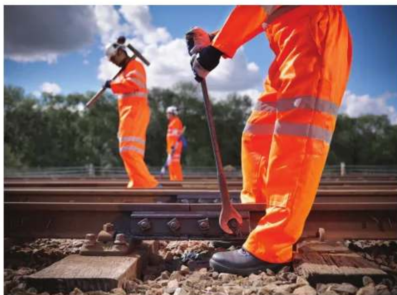
Figure 8 This worker uses a long wrench because it requires him to exert less force to tighten and loosen the nut. The wrench has a long lever arm, and less force is required if the force is applied farther from the axis of rotation (the center of the nut).
