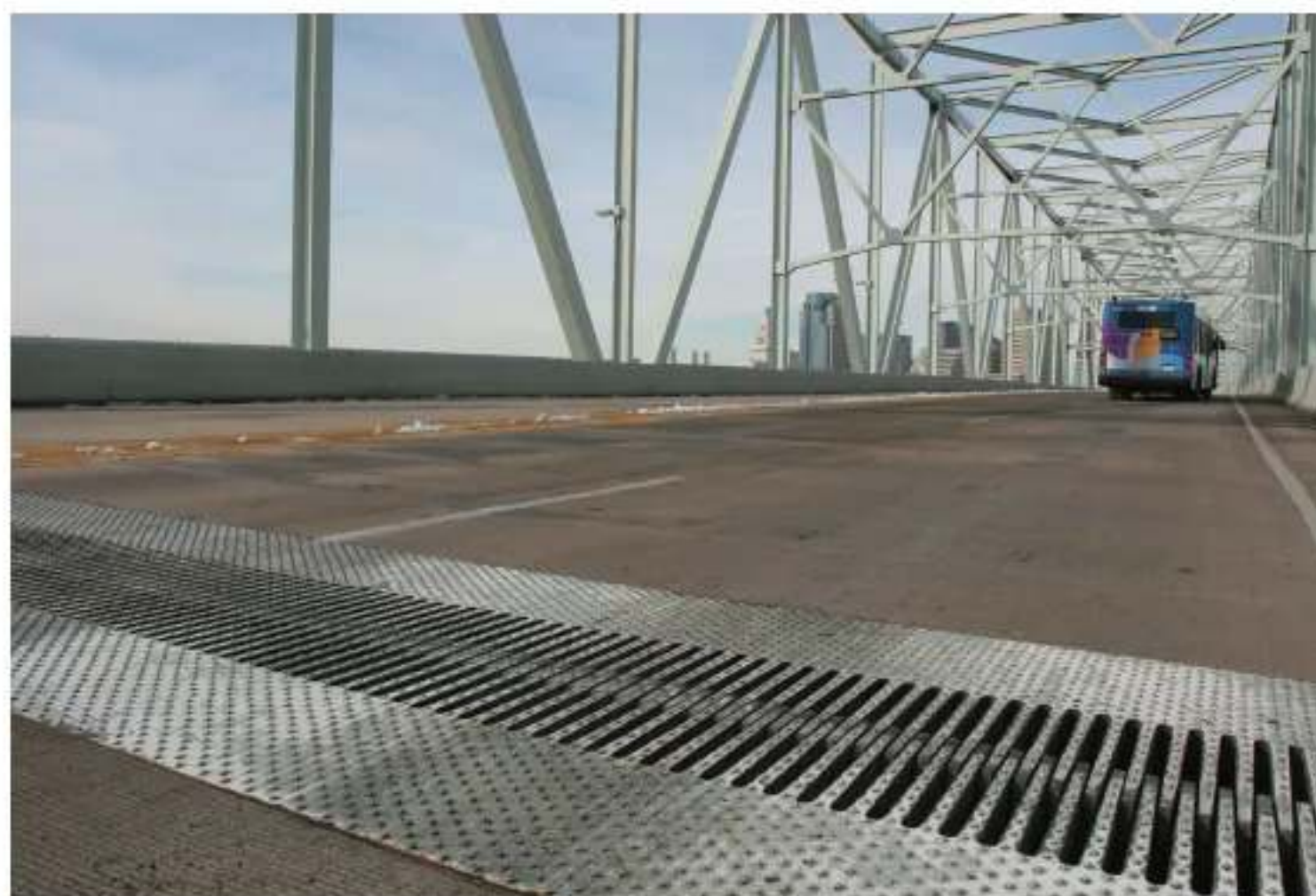
Figure 20 Expansion joints are included when bridges, roads, and train tracks are built.
