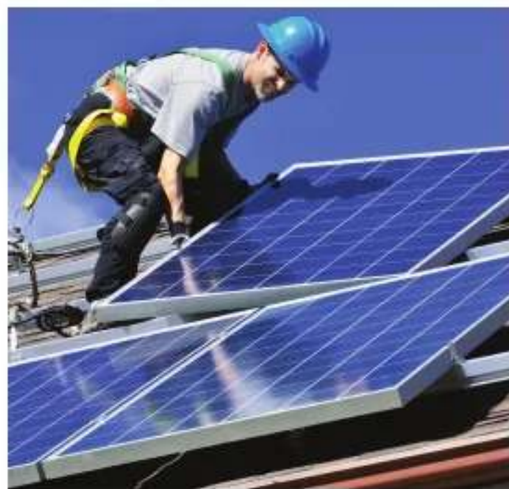
Solar photovoltaic panel installer
