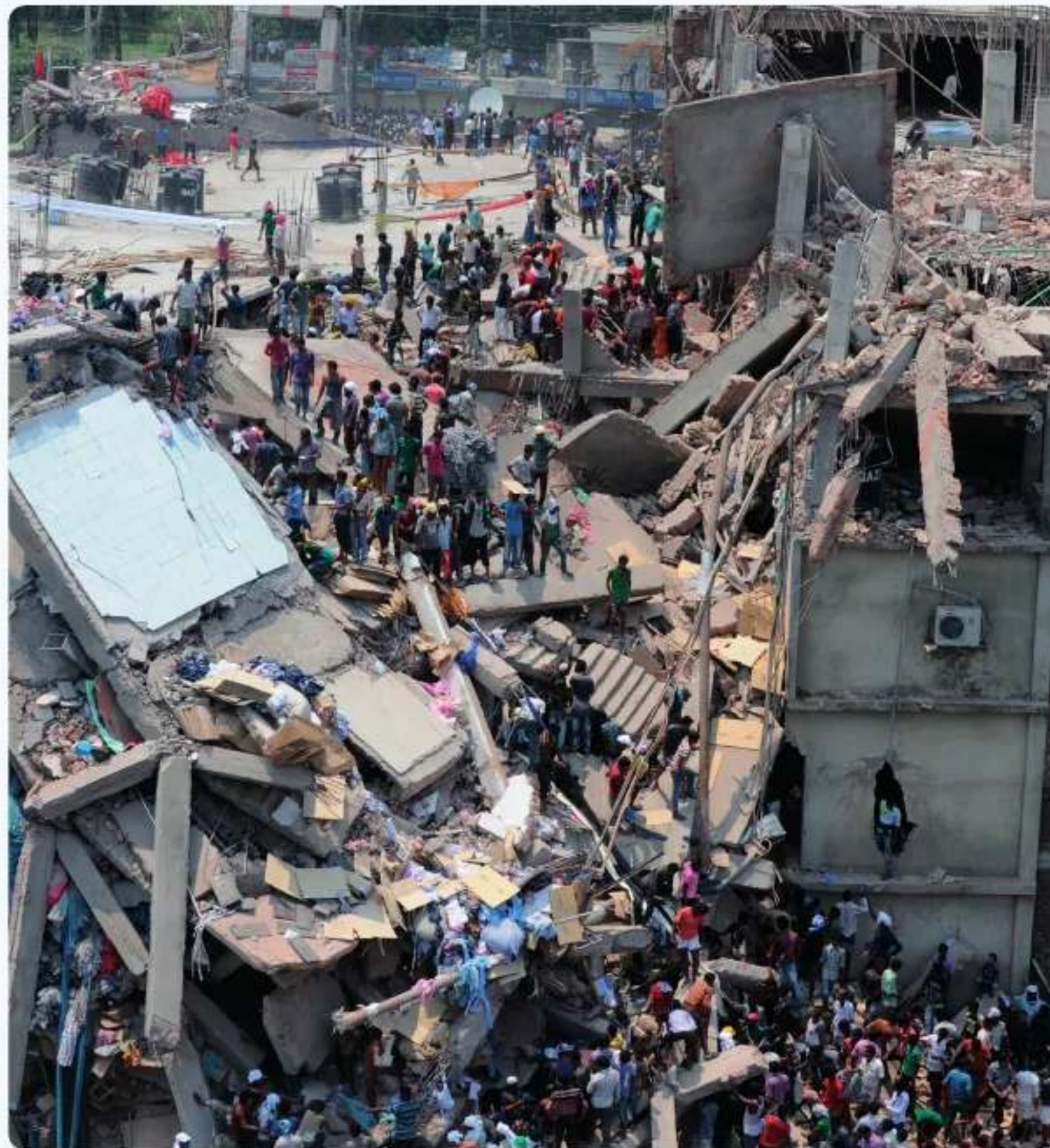
The Rana Plaza building in Dhaka on the outskirts of Bangladesh. Poor construction, inappropriate use and poor safety features contributed to the death of over a thousand people when it collapsed in April 2013.
